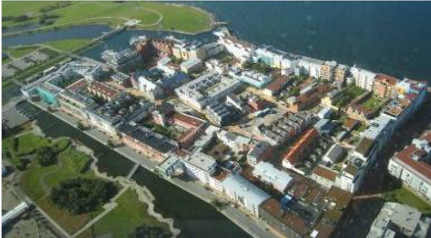
Western harbour/ Bo 01 Malmö
